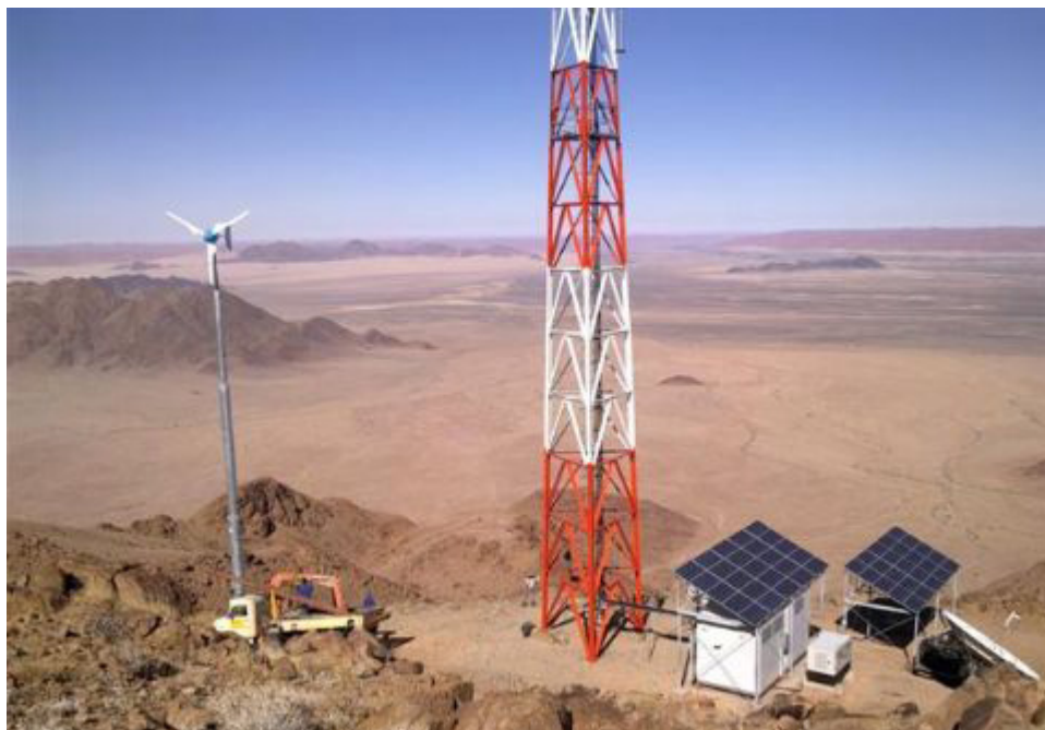
Figure 10. Hybrid wind-solar system for telecommunication tower (3 kW wind + 48 V PV), installed in 2010
