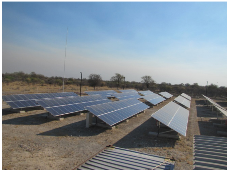
Figure 13. Solar panels at Tsumkwe
