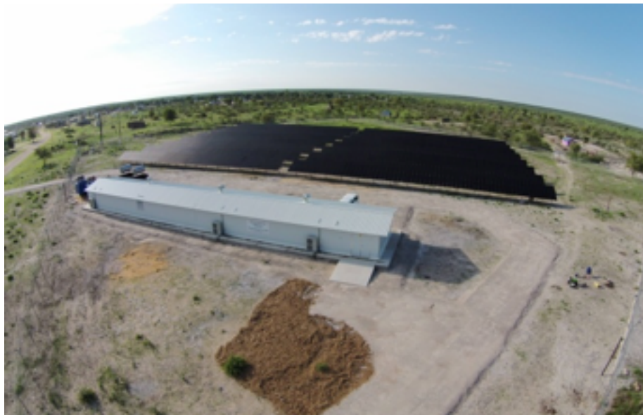
Figure 15. Solar panels at Gam
